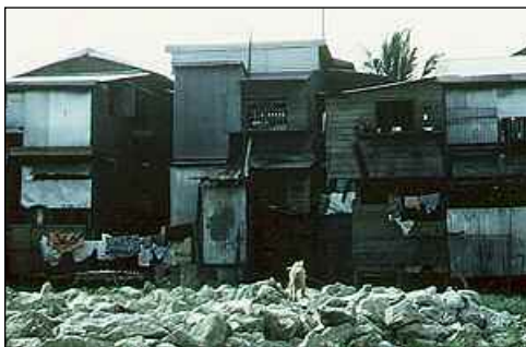
Shanty construction, Philippines
